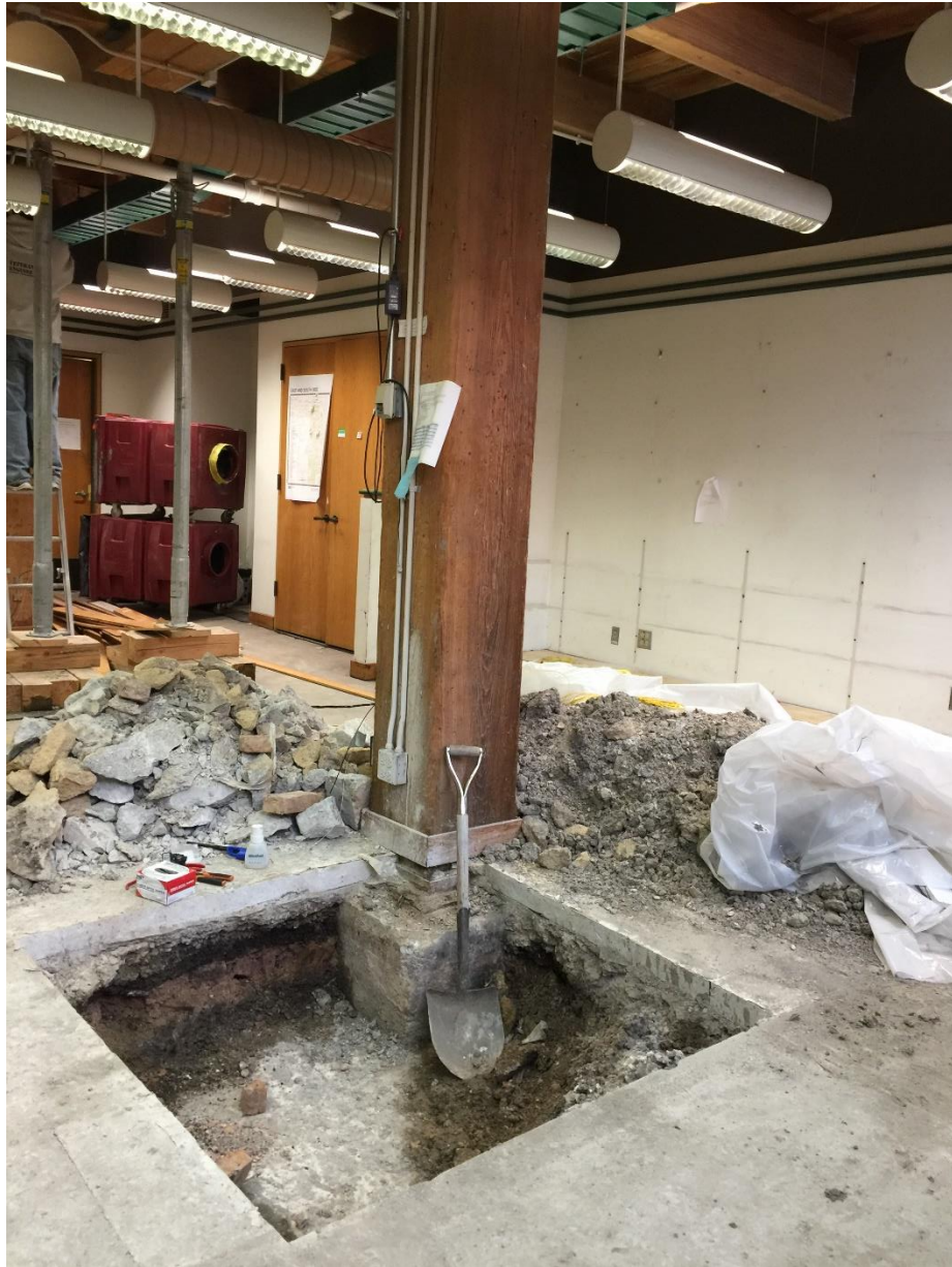
Figure 32. Typical timber column's footing
