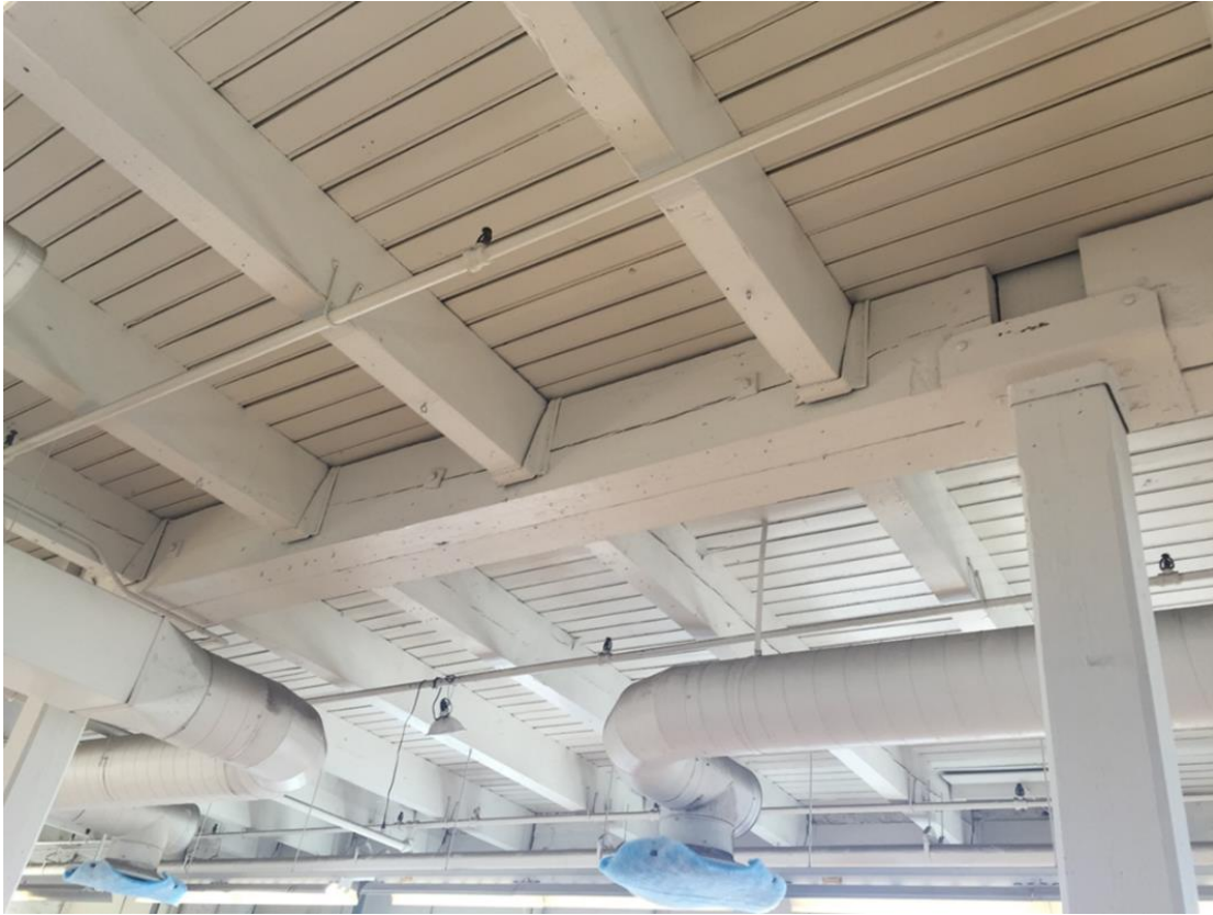
Figure 31. Timber structural system
