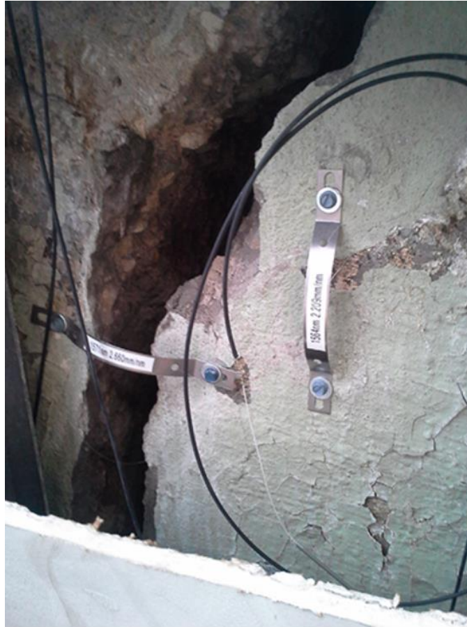
Figure 35. Typical cracks in the masonry wall as a result of differential settlements
