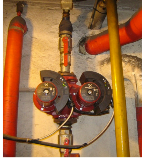
Figure 8: Twin pump number 2 (recently replaced)
