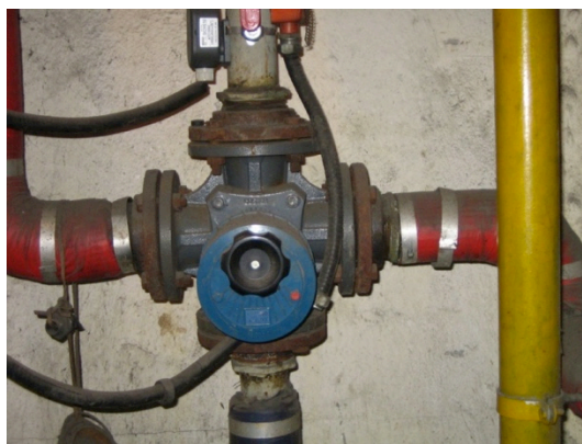
Figure 6: Four-ways mixing valve
