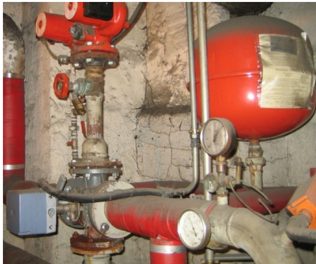
Figure 11: Expansion tank boiler
