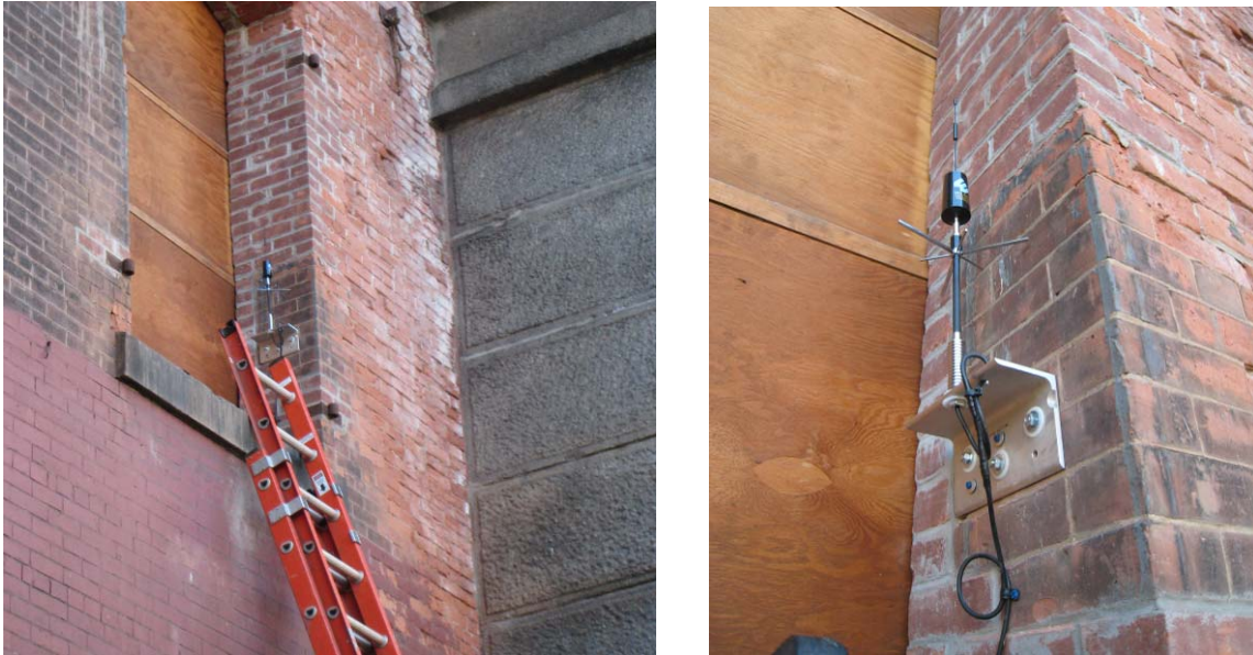
Figure 27. Cellular antenna installation.
