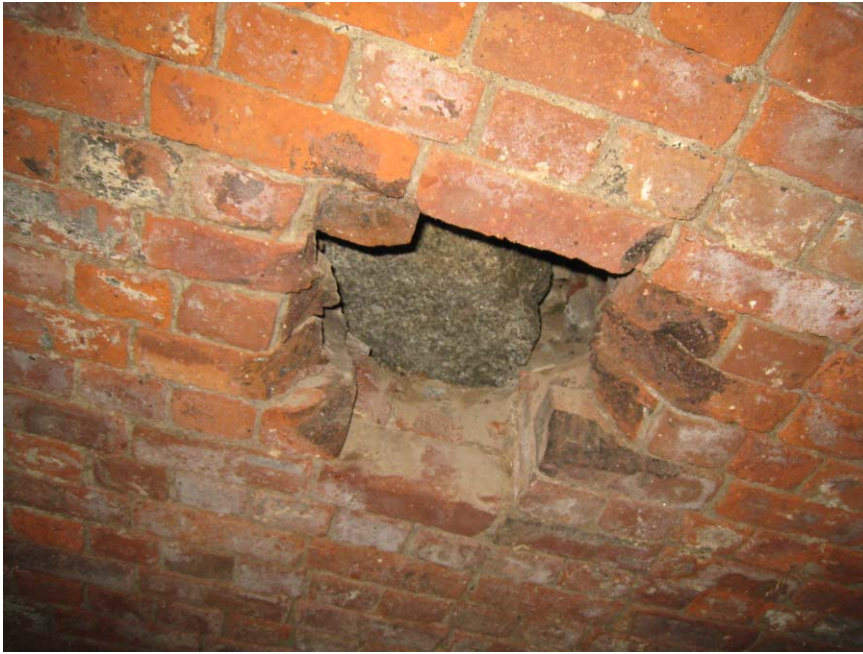
Figure 21. Inspection opening in arch showing 2' brick thickness and granite rubble fill.
