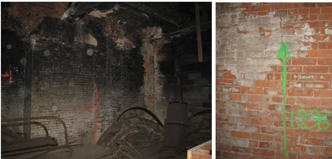
Figure 20. Vertical masonry cracks indicating past differential settlement.
