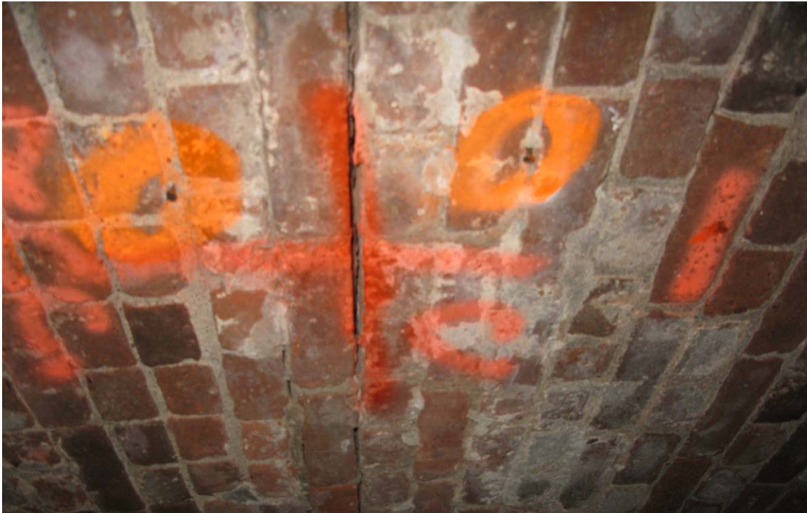
Figure 19. Longitudinal crack at the crown of the arch.
