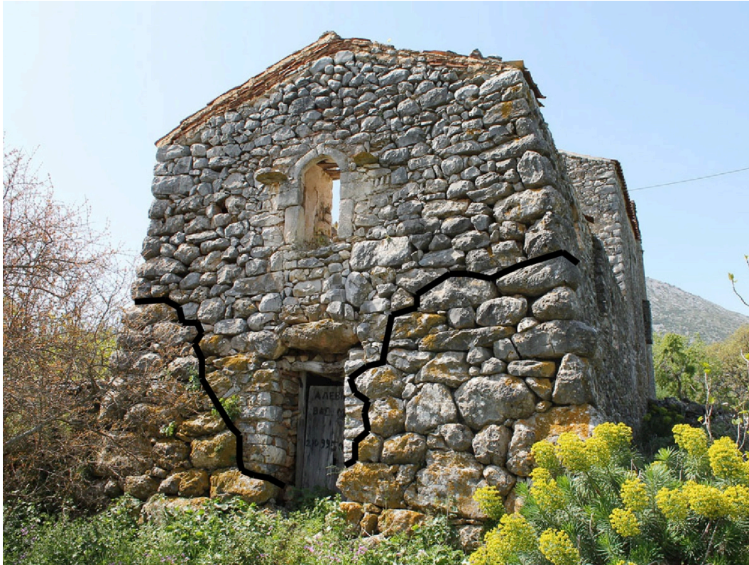
Figure 6. Megalithic house with Ottoman II reconstruction in Chimara (T029F005). The black line shows the approximate division between the two phases of construction.
