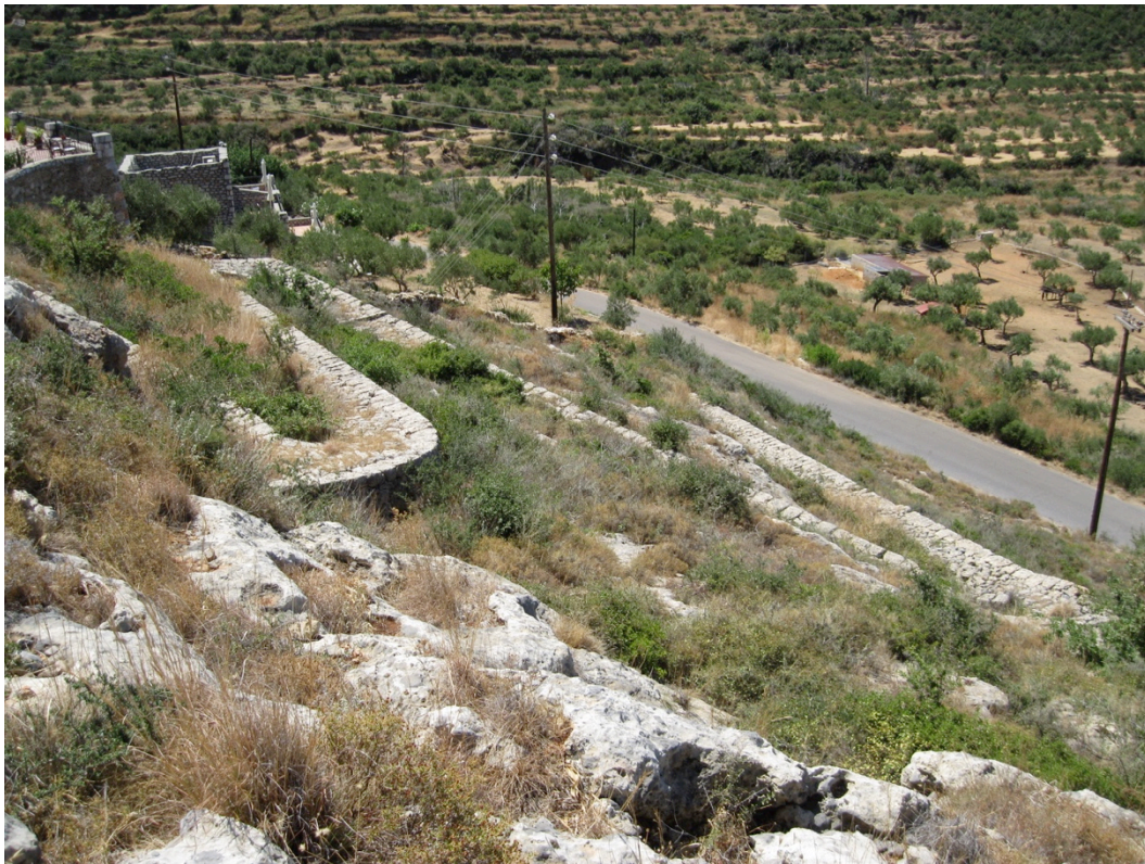
Figure 34. Kalderimi leading downhill from the Ottoman fortress of Kelepha, showing Z-shaped turns (K0029S08).
