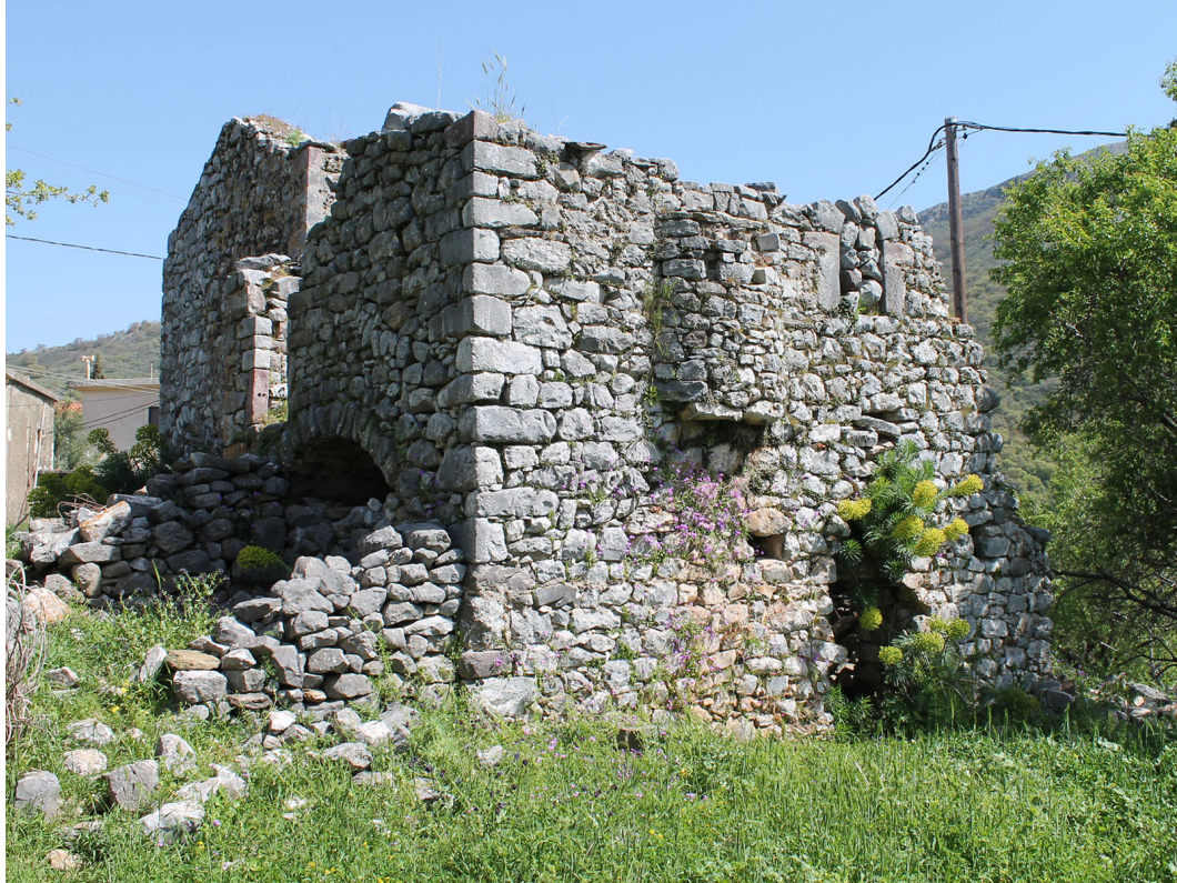
Figure 13. Residential structure in Chimara showing typical Ottoman II-period construction, with gabled roof, second-floor doorway accessed by a stairway, a ground floor kamara (just below doorway), arched windows, and a defensive klouvi (T029F004).
