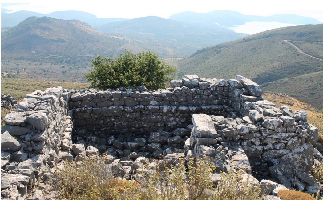
Figure 159. Palaia Tserova: Typical Ottoman-I residential structure at the site, showing regular coursing and an intact ledge for supporting floor beams (T301F005).
