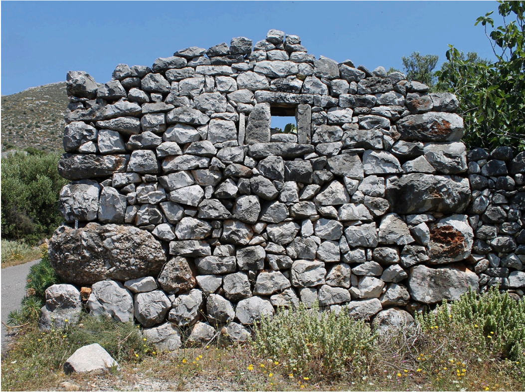
Figure 12. Residential structure in Diporo showing typical Ottoman I-period construction, with megalithic cornerstones and a small window on the narrow end (T034F009).
