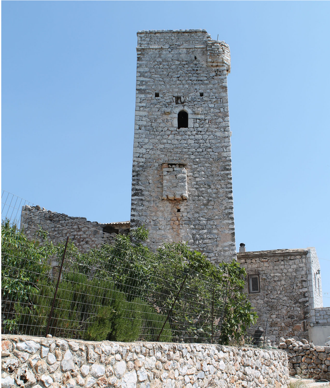
Figure 14. Post-Ottoman tower in Briki, with a petromachos protecting the third-story window, polemotrypes above fourth story, and a klouvi projecting from the roof (T024F026).
