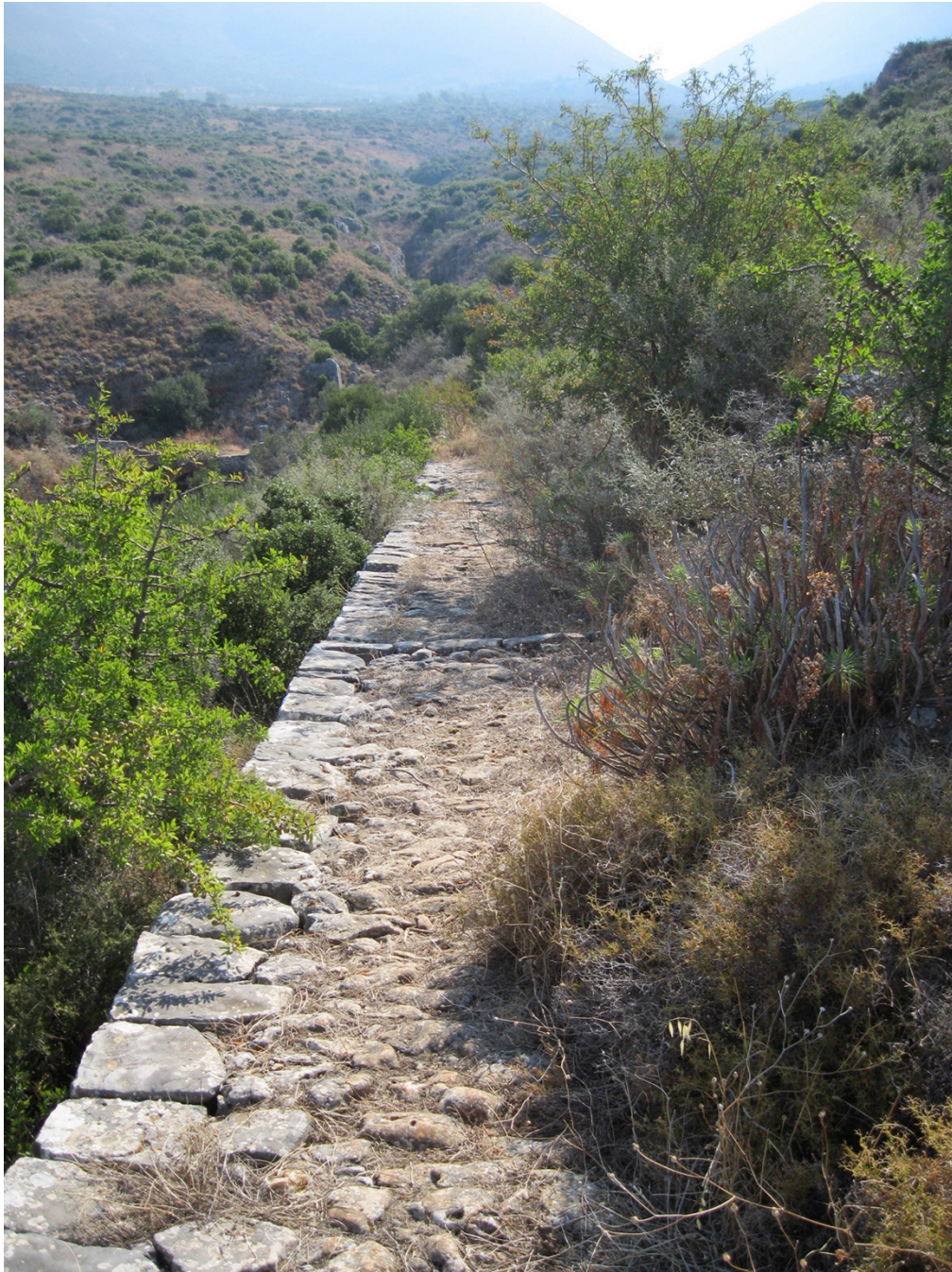
Figure 149. Long-distance kalderimi connecting Pyrgos Dirou and Areopoli (K0016S01). Note the left edge is built up substantially from the ground below to create an even platform.
