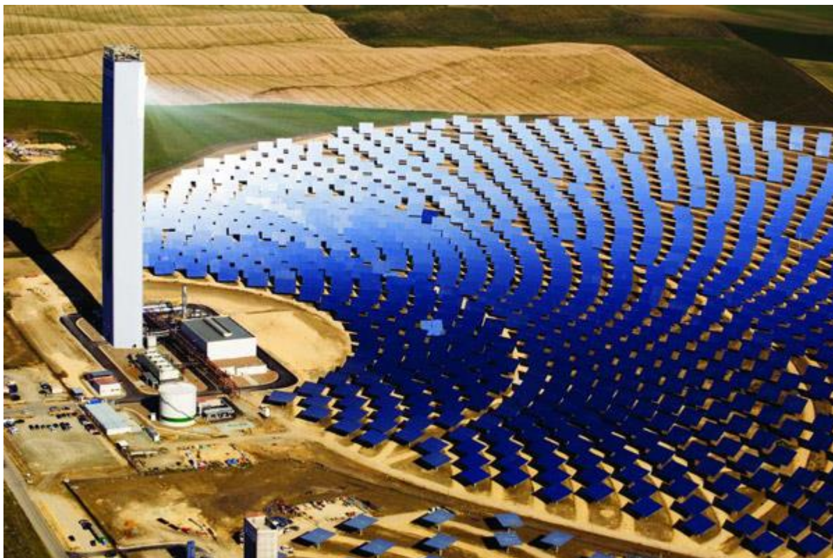
Figure 6: Example of solar field on the polar side of the tower [29]
