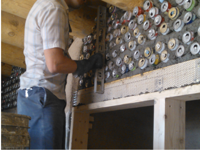
Figure 13. Construction of Can Wall (Personal Photo July 2014 Taos, NM).
