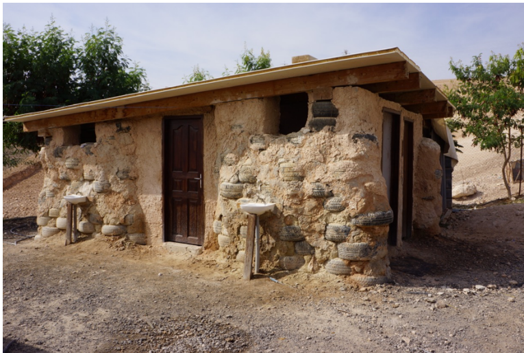
Figure 10. Tire construction in Palestine (Clarno 2012).
