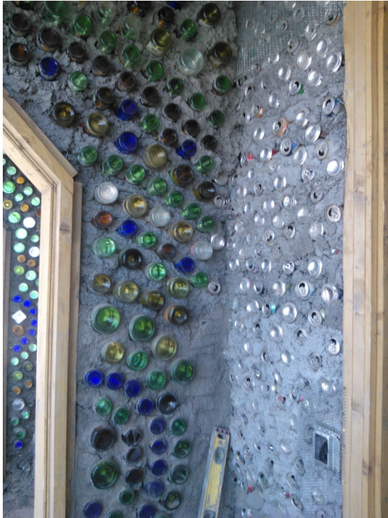
Figure 14. Bottle wall under Construction (Personal Photo July 2014 Taos, NM).
