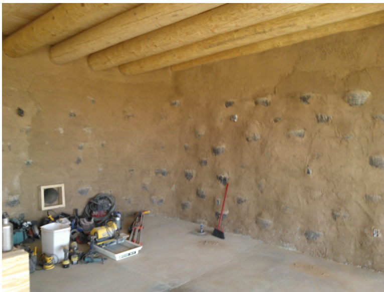
Figure 11. Interior tire wall (Personal Photo July 2014 Taos, NM).
