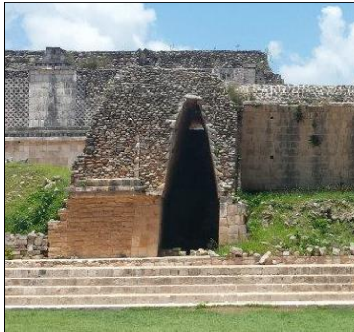
Figure 2.13 Uxmal, Mexico. Stone vaulting with "boot-shaped" construction stones. Author's photograph, July 2014.
