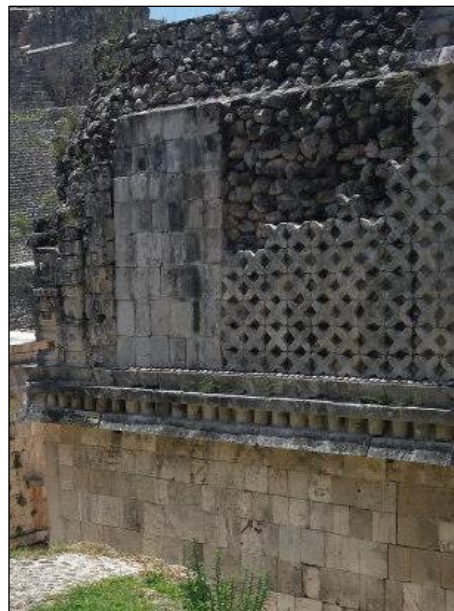
Figure 2.14 Uxmal, Mexico. Evidence of a rubble core faced with cut stone. Author's photograph, July 2014
